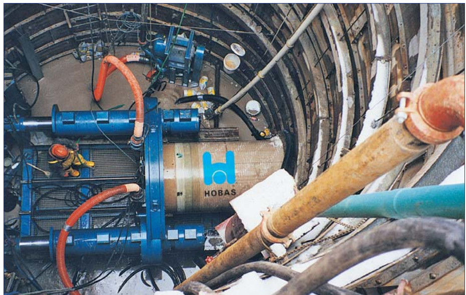
HOBAS pipe is well accepted in Hawaii and is being used for several microtunneling projects in both Honolulu and Maui counties.
