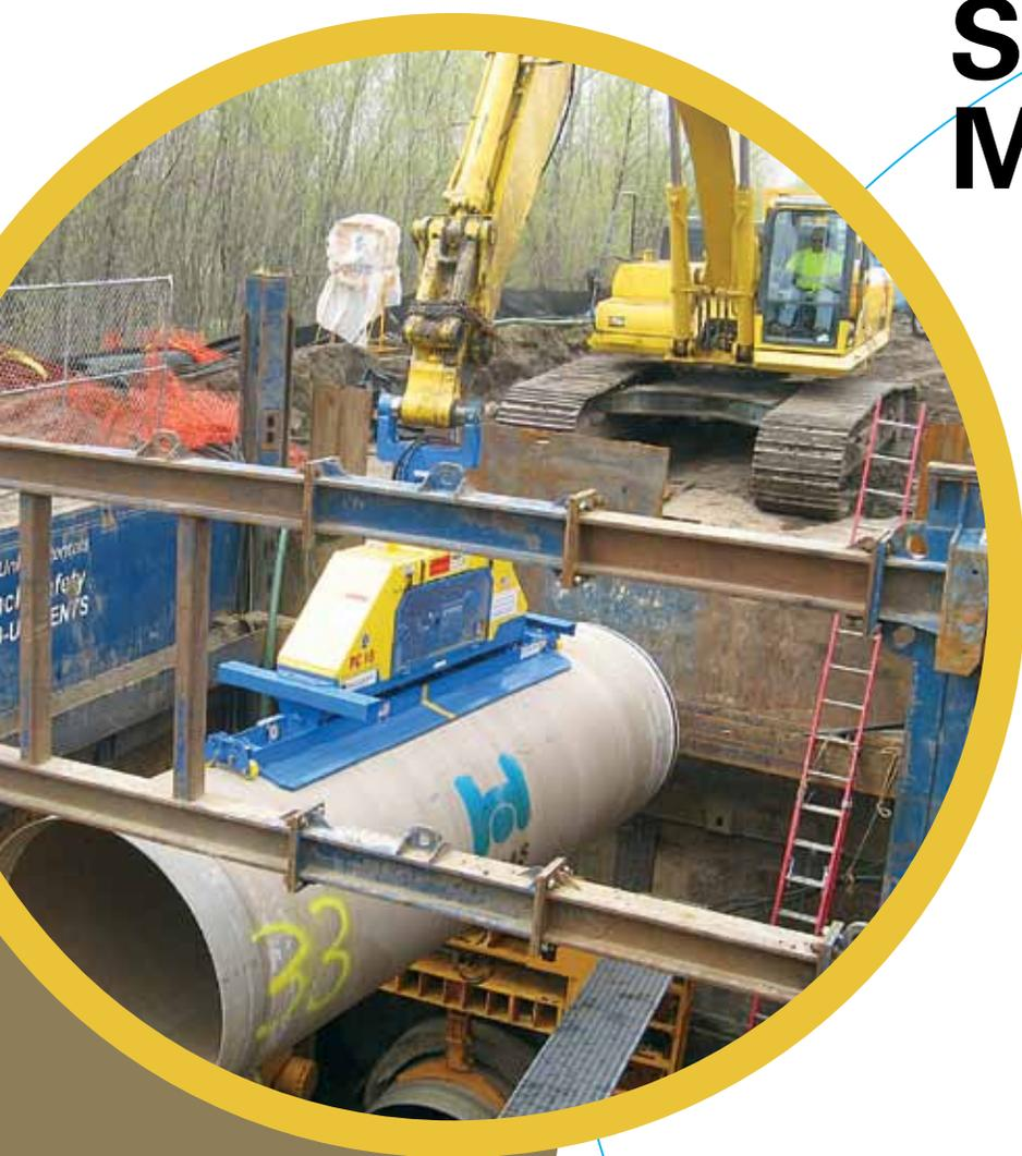
Light weight CCFRPM can be handled with minimal equipment. Here a 66-inch large diameter pipe is lowered into an installation pit.
