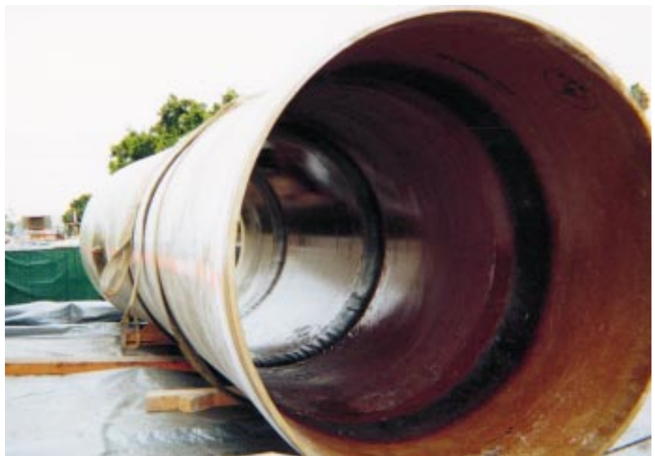
Radius fittings were manufactured on site to match existing sewer alignment.
