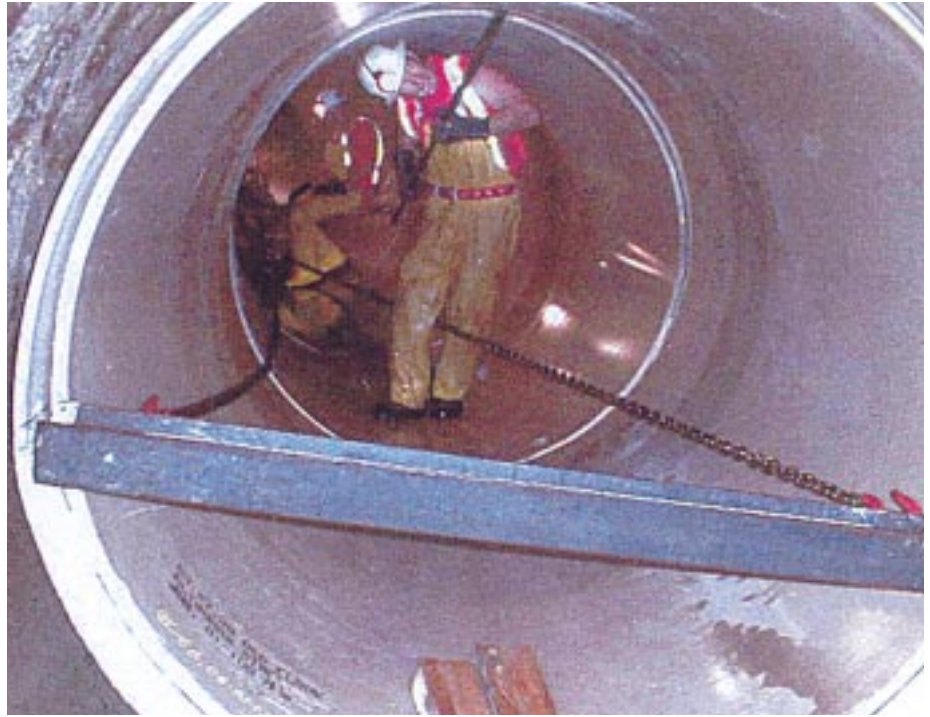
Pipes were joined in the curve using a winch.
