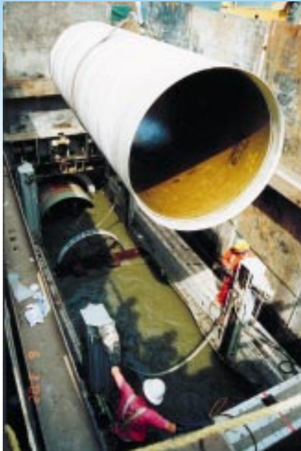
Gasket sealed HOBAS Pipes do not require bypass pumping.
