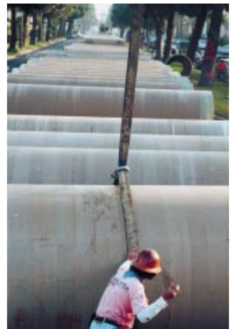
Sliplining progressed rapidly achieving rates of 5 minutes per pipe.
