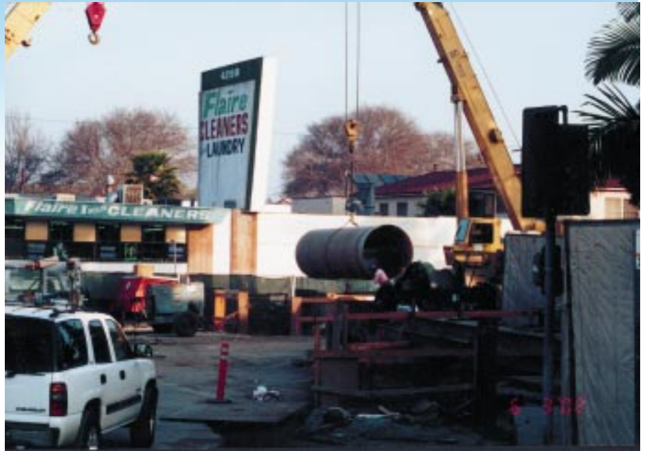
Buntich sliplined sections of sewer which traveled under homes and businesses.
