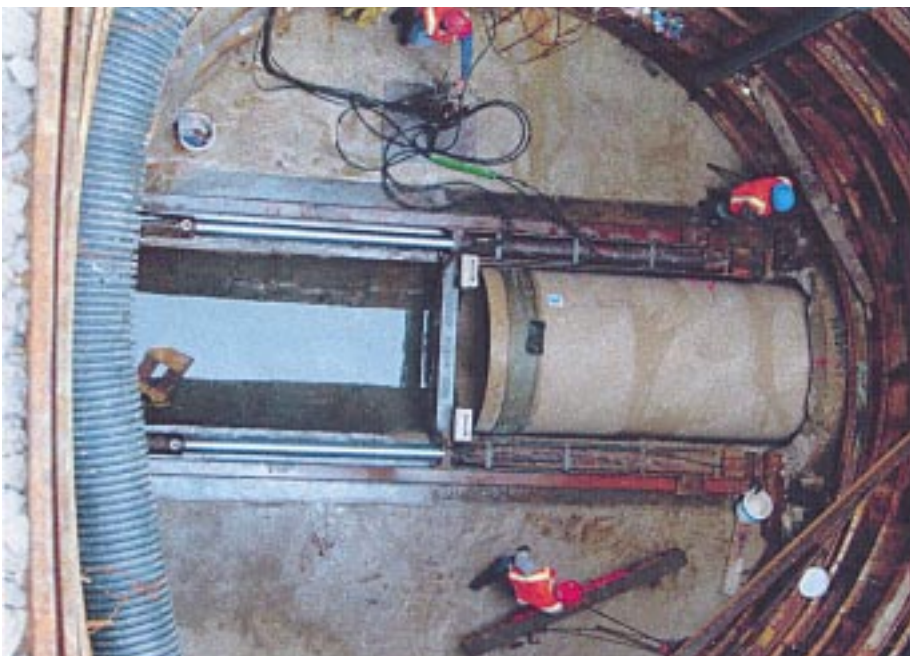
The 66" pipe was pushed through the 72" deteriorated concrete line.
