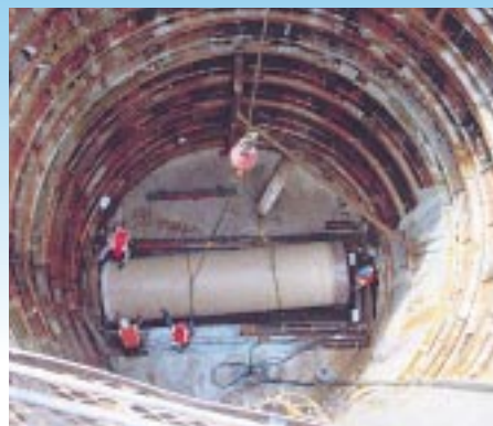
Lightweight segmental sections are strong enough to handle 70 foot depths.
