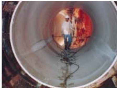
The high strength pipe wall allowed for a smaller primary tunnel.
