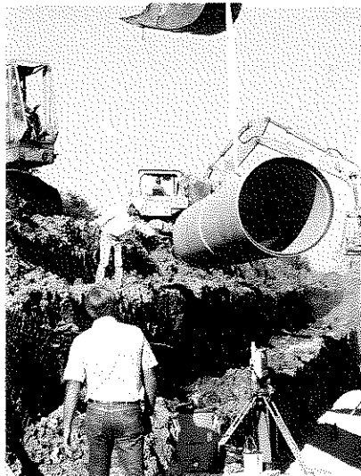
20 ft. long Hobas USA pipe weighing 2500 lbs. being lowered into the trench with a 235 backhoe.
