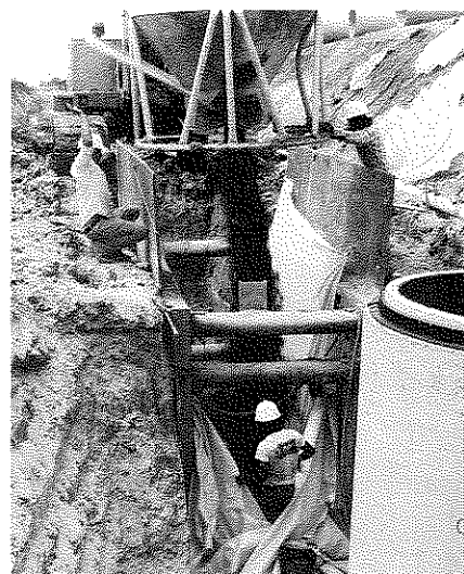
42" Hobas USA pipe installation in trench box construction.
