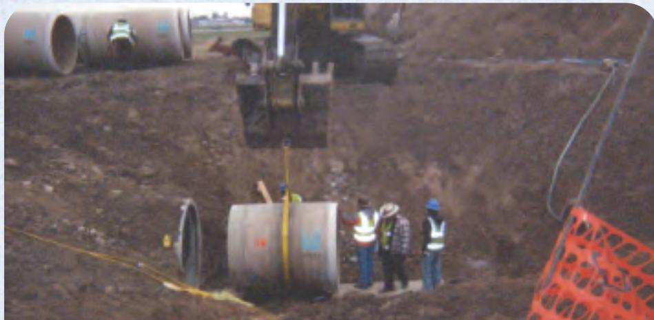
HOBAS PROVIDED MITERED FITTINGS TO EXACTLY FIT THE ALIGNMENT OF THE EXISTING WATERLINE UNDER RUNWAY 13/31.
