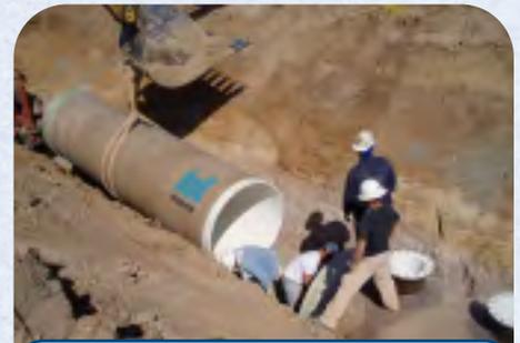
LIGHTWEIGHT HOBAS PIPES WERE QUICKLY AND SIMPLY INSTALLED. PUSH-TOGETHER COUPLINGS SPEED INSTALLATION.
