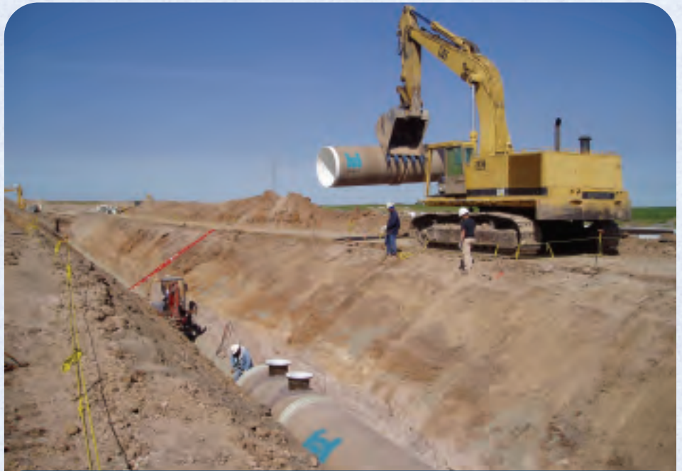
HOBAS MANUFACTURED SEVERAL FITTINGS INCLUDING THIS 60-INCH DIAMETER TEE FOR OVERAA CONSTRUCTION TO USE ON THE SOUTH SAN JOAQUIN WATER TREATMENT PLANT PROJECT.
