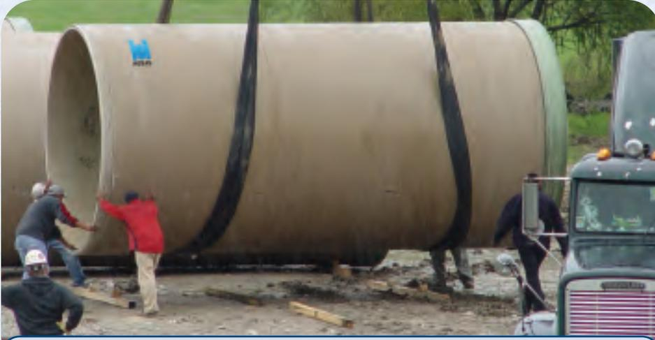
HIGH STRENGTH AND DURABLE, HOBAS CCFRPM IS ALSO LIGHT-WEIGHT COMPARED TO MANY ALTERNATIVE PRODUCTS
