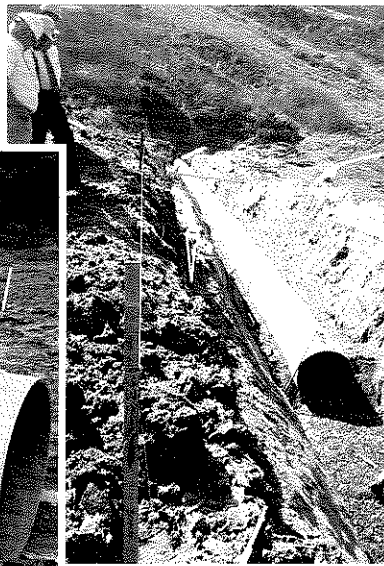
36" direct bury installation
