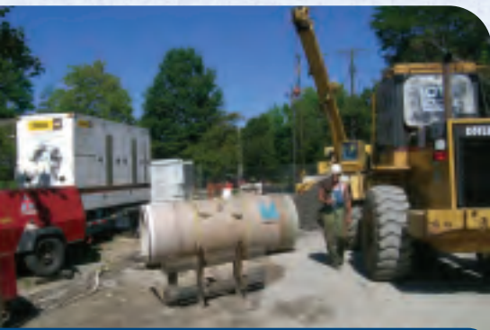
A 10-FOOT SECTION OF HOBAS PIPE AWAITS INSTALLATION.
