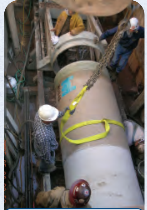
JACKING RUNS RANGED FROM 460 TO 700 FEET FOR THE 36-INCH PIPE.
