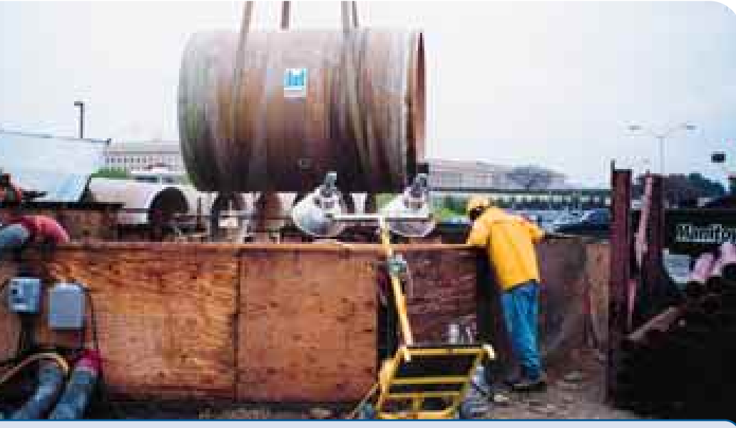
HOBAS PIPES WERE LIGHTER THAN THE CONCRETE ALTERNATIVE.
