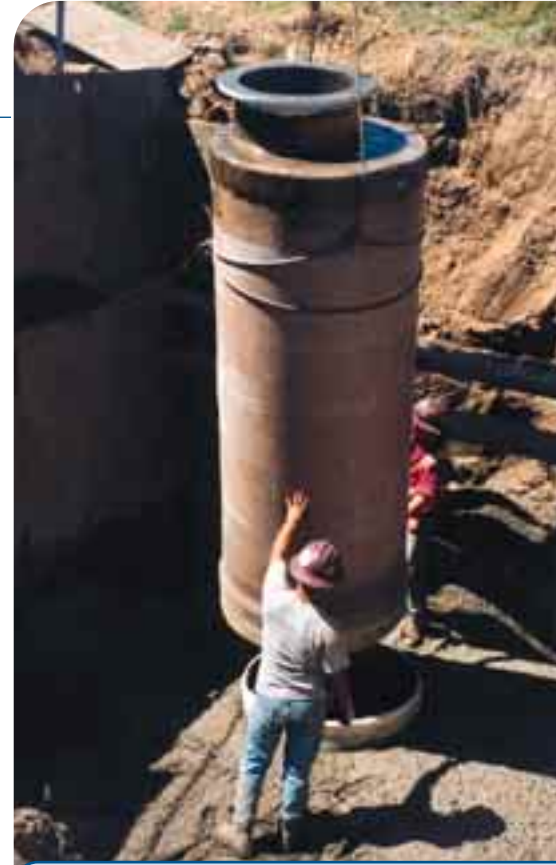
THE HOBAS RISERS WERE SIMPLY ATTACHED WITH AN FWC COUPLING.
