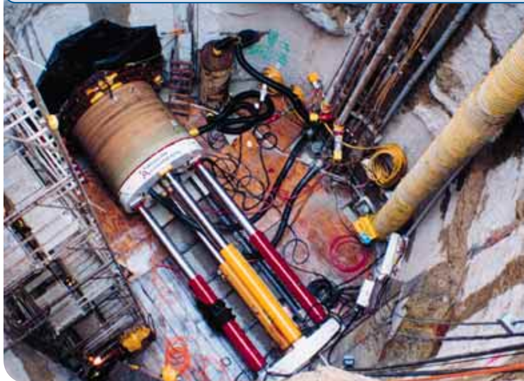
SMOOTH NON POROUS OD OF THE HOBAS PIPE CREATES LESS FRICTION.
