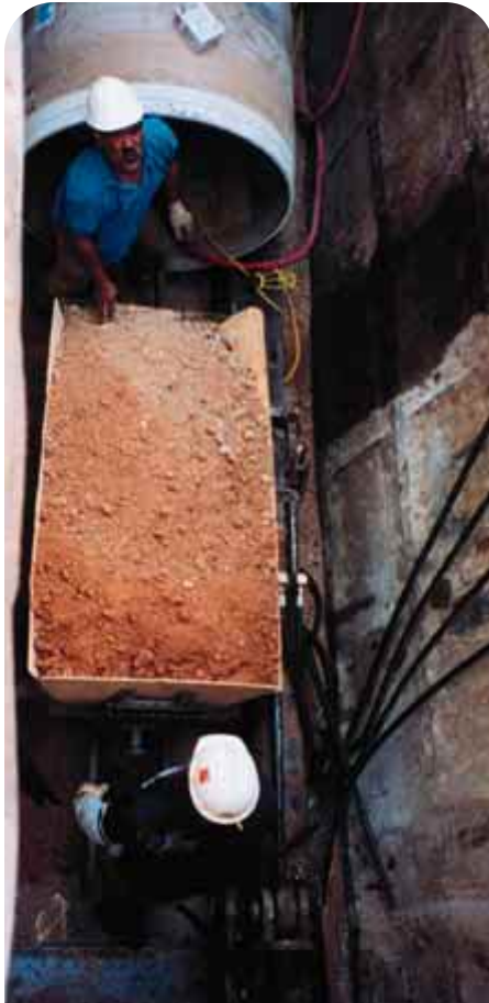
SPOIL WAS REMOVED FROM THE TUNNEL VIA MAN RIDDEN CARS, AND A RAIL SYSTEM ON THE INTERIOR OF THE HOBAS PIPES.
