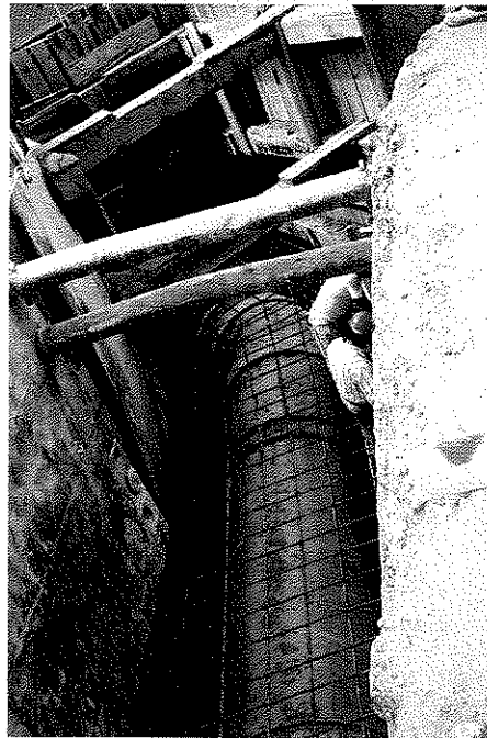
Reinforced encasement at elbow provides economical thrust restraint
