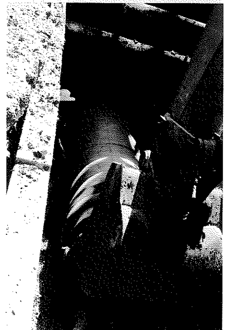
Fast insertion of Hobas pressure pipe into the bore hole
